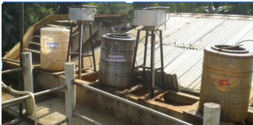
Figure 5 A custom designed Arsiron Nilogon dosing unit at Jyotinagar Public Water Supply Scheme which worked for over 5 years in Golaghat, Assam, India.
