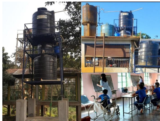
Figure 3 Two 1000L small community filter which remove neurotoxic Mn, Hg and Pd along with Fe from drinking water to children with neurological issues at MRC in Assam
